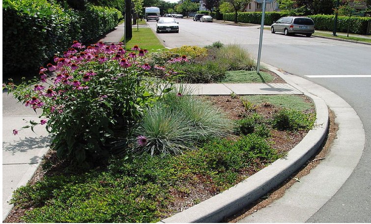
FIGURE 9: CURB EXTENSION (SOURCE: CITY OF VANCOUVER)
