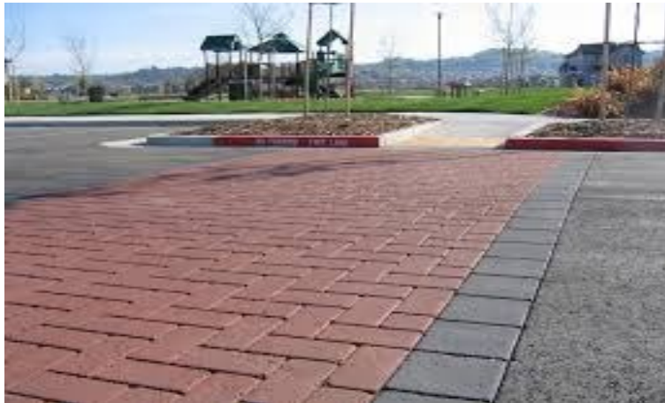
FIGURE 5: TEXTURED CROSSWALK (SOURCE: STREETPAINT.COM)
