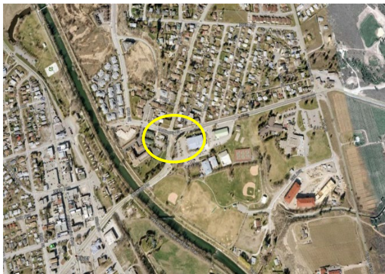
FIGURE 45: SITE OVERVIEW KIWANIS PARKS AND RECREATION AT PARK DRIVE
