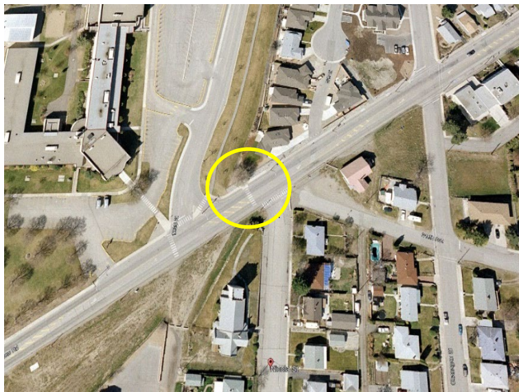
FIGURE 38: INTERSECTION OF FAIRVIEW ROAD AND NICOLA STREET
